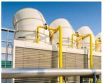
Eco-Clean Dosing in Cooling Towers to reduce frequency of blow down
